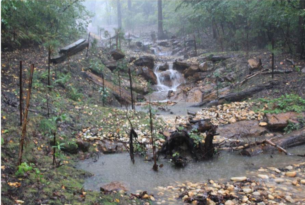
Photo 11: Example of boulder cascade channel stabilization.
