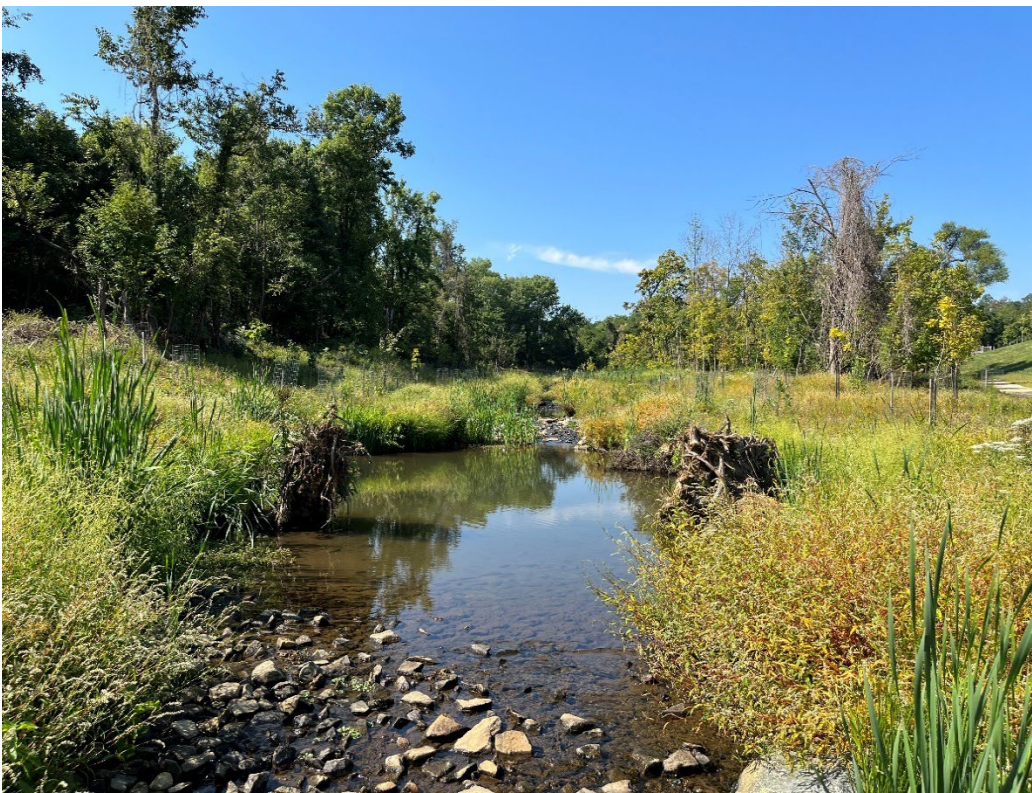
Photo 15: Example of riffle pool restoration with floodplain reconnection and large woody debris installations.
