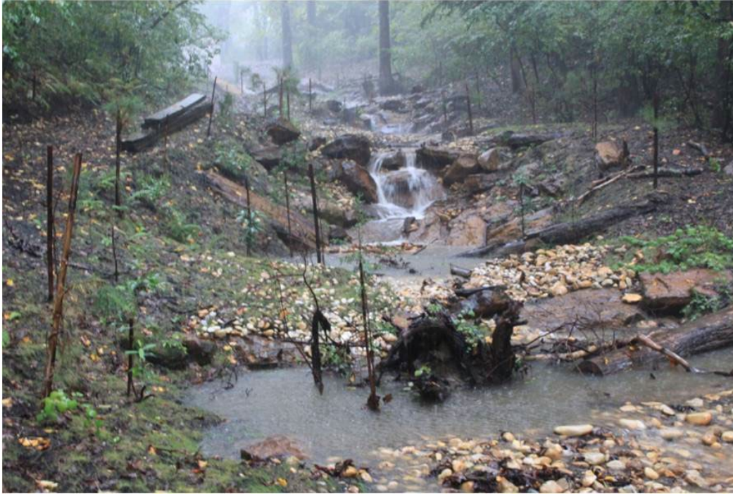
Photo 11: Example of boulder cascade channel stabilization.
