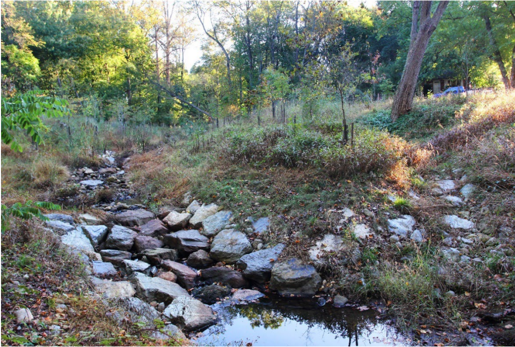
Photo 10: Example of boulder cascade channel stabilization.
