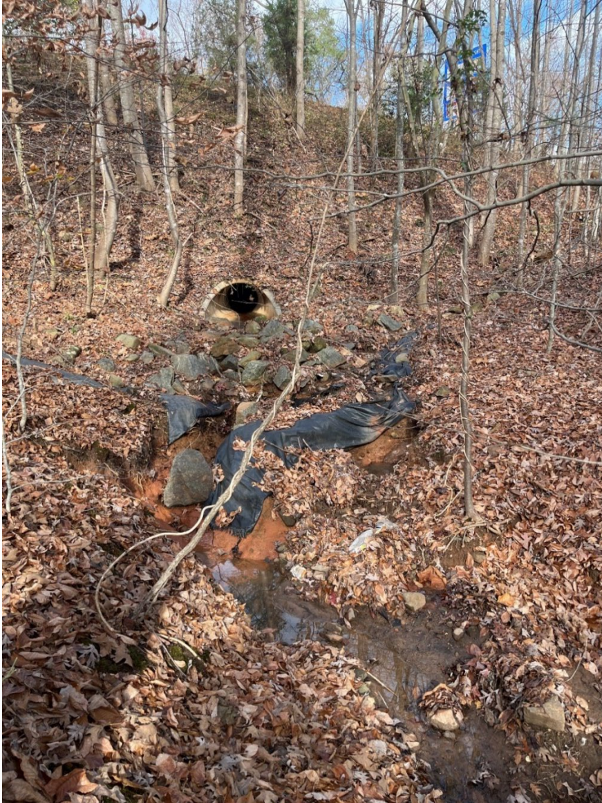
Photo 1: Headcut at Reach 1 outfall.
