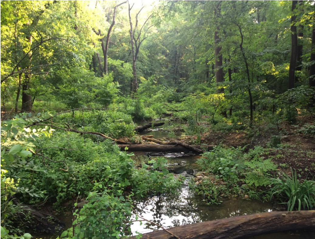
Photo 13: Example of riffle pool restoration with incorporated large woody debris with raise in channel bed and bank grading.
