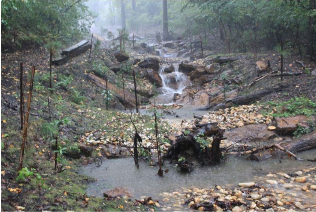
Photo 11: Example of boulder cascade channel stabilization.
