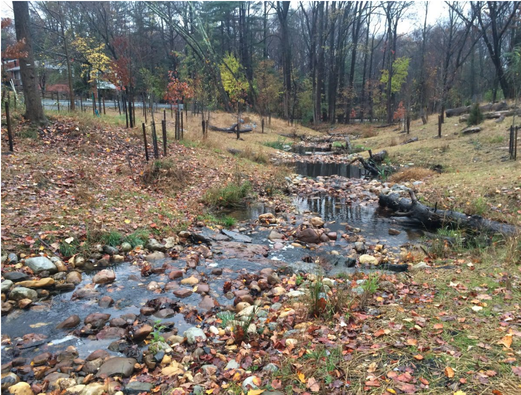
Photo 12: Example of riffle pool restoration with raise in channel bed and bank grading.
