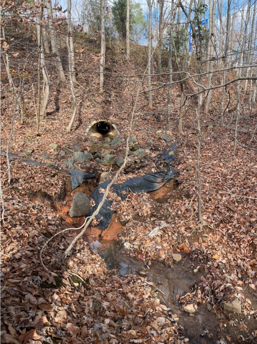
Photo 1: Headcut at Reach 1 outfall.
