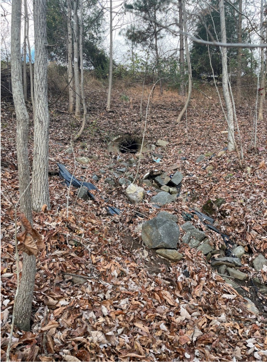
Photo 2: Headcut at Reach 2 outfall.
