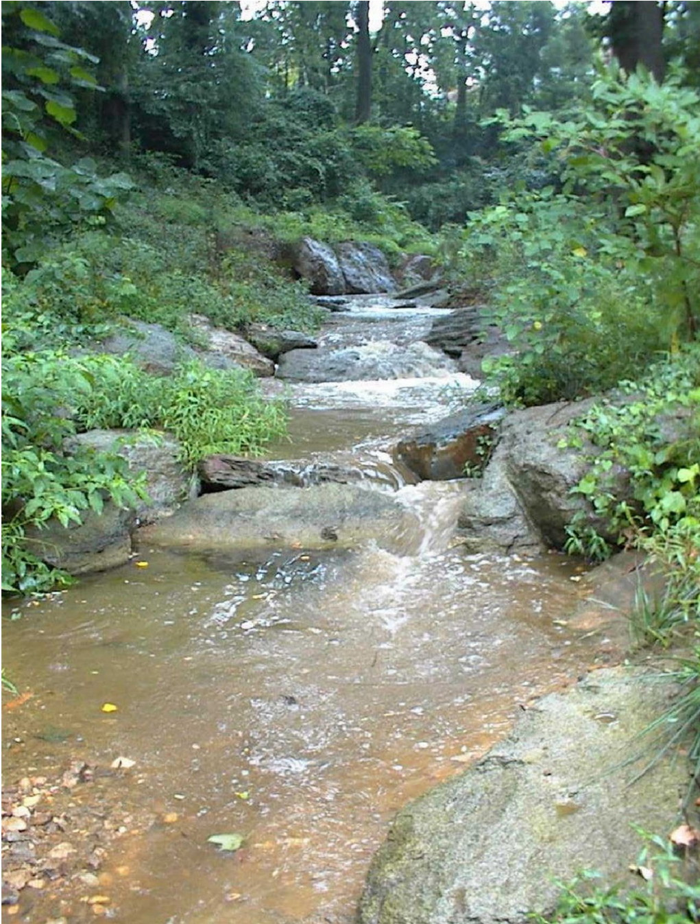
Photo 14: Example of cascade pool restoration with raise in channel bed and bank grading.
