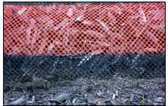
Close Up of Sediment Control
